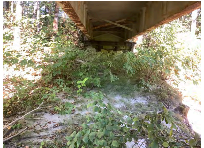
Right Bank Abutment when facing downstream
