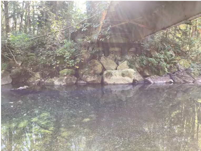
Left Bank Abutment when facing downstream
