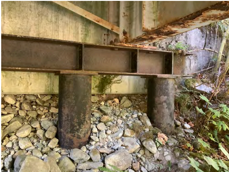
Left Bank Abutment when facing downstream
